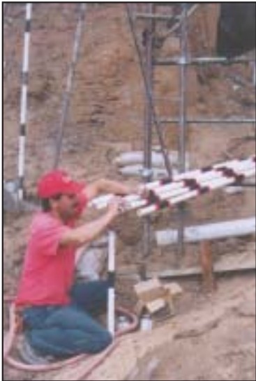
20,000 LF - Dana Point, CA project
